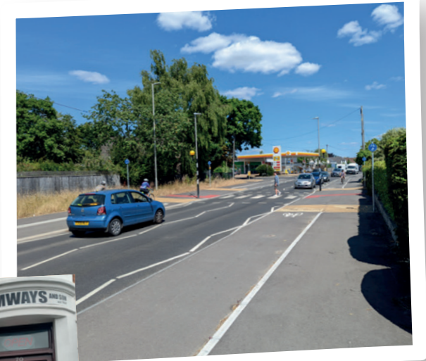
New walking and cycling paths and parallel crossing on Leigh Road and Wimborne Road West from Wimborne to Colehill / Canford Bottom.
