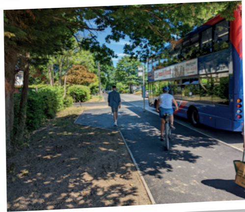
The new shared cycling and walking path, and bus stop improvements on Ringwood Road, Ferndown.
